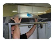
If any drilling is required, the Steam Stopper product can be drilled with any standard drill bit. The best results are achieved without the use of a pilot hole.
