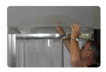
Now simply slide the Steam Stopper onto your Shower and into the U-channels. No fixing of the Steam Stopper product to the top of your shower is required.
